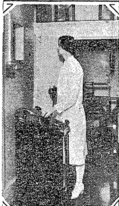
TRANSFORMER AND CONTROL BOARD
