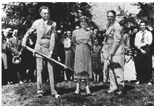
C. C., Mabel and Neil Criss breaking ground for the Mutual of Omaha Building
